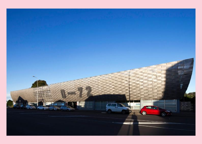
Completed in 1996 D72 was designed by Patterson Architects using a woven aluminium façade to filter New Zealand's bright sunlight.
