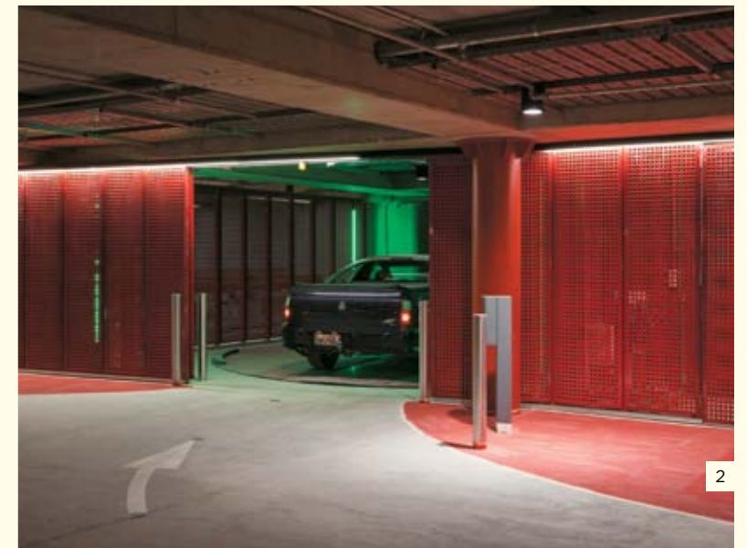
1. Interior view showing penetration of natural light through the twin façade at Geyser, in Parnell. 2. The building's automated car stacker in action.
